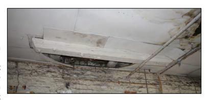
it was intended as a long-term fixture, bolted from the floor above at either end. Possibly relates the hanging of a short line shaft or pulley associated with the hoist inserted into the southern part of the bay (5/14).
