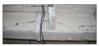
drum or roller, as it has an elongated run out at its southern side, more suggestive of being caused by a steel rope or possibly leather shafting belt.
