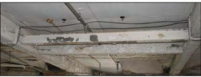
the south of timber beam 5/30 to the immediate north. The beam is fixed with square-headed bolts to either face at both ends, and is possibly associated with a pair of flitch plates on the soffit of the western ceiling beam (5/32) to the south. It blocks what appears to be a drum scar (5/33) on the east face of the west beam, further suggesting a relatively late date of insertion.
