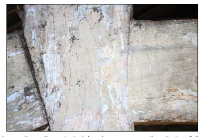
remains of a single 'I' is visible on the adjacent straining beam, suggesting that a full corresponding assembly mark survives beneath significant layers of paint
