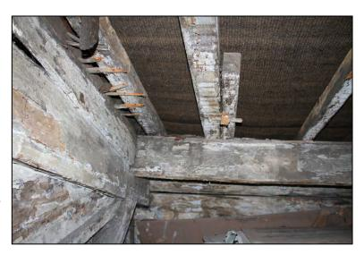
**Assessment of Significance:** The rafters appear to have been part of the original roof structure, but it is unclear whether they survive in their original position, or were simply reused during the refurbishment of the roof. However, they, are considered to be of HIGH significance, and should be retained during the roof repairs if practical. However, should this prove unfeasible, their loss has been mitigated by 3D laser scanning and photographic recording.
