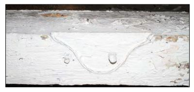
approximately <sup>3</sup>/<sub>4</sub>" depth. It has a solitary bolt thread protruding from its southern end, and probably formed the base of an L-shaped bracket attached to the beam. Similar style and size to feature *5*/17, located on the same beam to the north.
