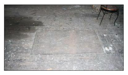
**Assessment of Significance:** Whilst the metal plate signifies the redundancy of the original power transmission system, it is probably of relatively early date, and is therefore considered to be of MEDIUM significance. It's retention is not critical to the future visual interpretation of the attic space, so long as the aperture it covers is not concealed without evidence for its position, for example, by a continuous floor covering.
