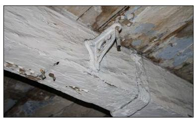
(5/39) has been retained following the removal of the remainder of the sprinkler system. As the only extant evidence of this important feature, it is considered to be of MEDIUM significance.
