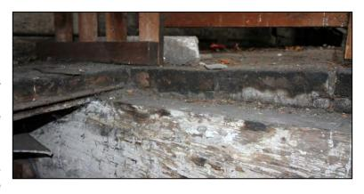
typically  $10\frac{1}{4}$ " wide and  $2\frac{3}{4}$ " thick, with 2" wide,  $\frac{1}{4}$ " thick metal tongue jointing them together. Similar boards are placed perpendicular within the eaves, although many have perished due to water ingress.
