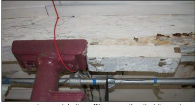
square-headed bolts. It has a wide compression mark in its soffit, suggesting that it may have formed the pad between a post and the tie beam prior to the relocation of the main line shaft to the north of the column line, in line with bearing box 5/12.
