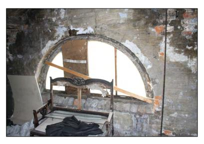
**Assessment of Significance:** The window apertures form an integral element of the structure and are of HIGH significance. Interventions should ideally be kept to a minimum to preserve this important original fabric. The frames and glazing are of little heritage merit.
