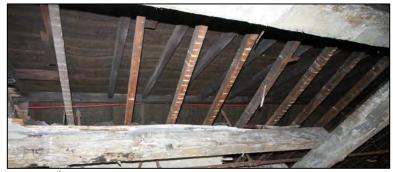
structures from the second half of the 19<sup>th</sup> century and more commonly associated with king post trusses. They appear to be butt-ended along the length of the roof, and form part of a renewal of the roof, that was probably associated with the addition of towers to the southern elevation of the mill in the early 20<sup>th</sup> century.
