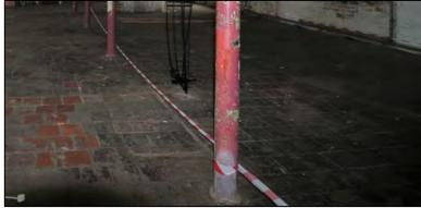
up layer above the curved brick arches of the floor below and appear to underly the column feet, suggest that they formed the original flooring of the mill. Their use within blocking of the original upright shaft bearing box suggest the re-use of salvaged tiles, rather than a complete reflooring of the whole floor a the time of the replacement of the original line shaft.
