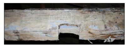
the northern part of the bay. Similar to that to the south (*5/51*) and overlain by hanger for sprinkler system, showing it to have been redundant by the early-20<sup>th</sup> century.
