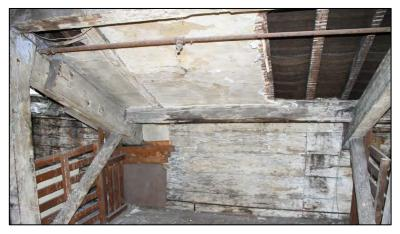
observed within Bays 1 and 2 (*6/14*), and to the northern eaves (*6/08*) being of a harder grey mortar, with charcoal rather than hair inclusions.
