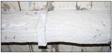
typical of a column headplate scar, possibly suggesting that there may have been an intention to replicate the two column rows seen on the floors below within the 5th floor. The scar is shallower than that to the north (5/42) but also covered by the stirrup between the tie beam and queen post of the truss above, demonstrating that the stirrups were not features of the original trusses, but were added subsequently.
