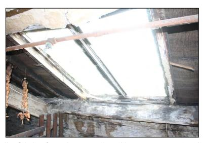
and central purlins and are typically of timber-framed construction, with narrow surround and glazing bar between the two vertical panes of later reinforced mesh glass.
