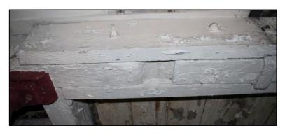
north, and became redundant following the strengthening of the tie beam with the addition of timber flitch plates *5/21*.
