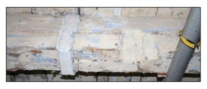
the bay. It has rounded ends, and is typical of a column headplate scar, possibly suggesting that there may have been an intention to replicate the two column rows seen on the floors below within the 5<sup>th</sup> floor. The scar is deeper than that to the north (*5/45*) and clearly covered by the stirrup between the tie beam and queen post of the truss above, demonstrating that the stirrups were not features of the original trusses, but were added subsequently.
