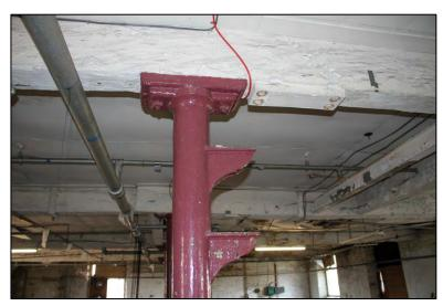
These appear to relate to line shaft hanger brackets, and are aligned with a 2ft wide bearing
