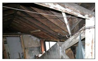
later remodelling, and that the refurbishment of the roof was taken significantly prior to 1928. It comprises common rafter rising to a ridge board, with a single slender hip purlin added at its angle with the south pitch of the main roof
