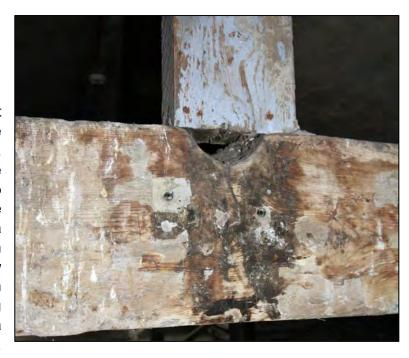
similar to the trusses to the east of the upright shaft. The cutaway is blocked by a king post inserted above the straining beam (6/13).
