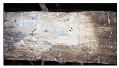
that were placed on top of each straining beam, carrying a line shaft down the length of the attic, in both directions from the upright shaft in Bay 3. That between Bays 1 and 2 also has a rounded cut out (6/12), possibly suggesting that the original intention had been to socket the bearing into the straining beam, rather than on a raised pillow bracket.
