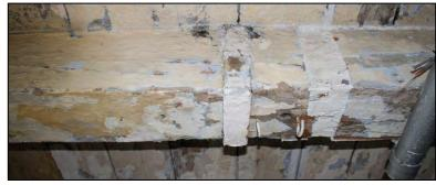
of the bay. It has rounded ends, and is typical of a column headplate scar, possibly suggesting that there may have been an intention to replicate the two column rows seen on the floors below within the 5<sup>th</sup> floor. The scar is clearly covered by the stirrup between the tie beam and queen post of the truss above, demonstrating that the stirrups were not features of the original trusses, but were added subsequently.
