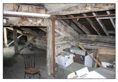
at its head feeding diminishing-section pipes throughout the attic. That providing the feed to the east blocks the line shaft position, demonstrating that this had become redundant by the time that the sprinkler system was installed.
