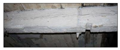
square section, placed at a slight angle to the beam, and is of unclear function, but is heavily painted, suggesting that it is not a modern feature.
