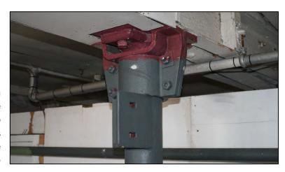
**Assessment of Significance:** This represents 20<sup>th</sup> century strengthening of the eastern tie beam, but detracts from the form of the highly unusual eastern column, possibly causing stress to the vertical casting for the end bearing of the original line shaft. It is therefore considered to be of LOW significance.
