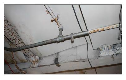
hangers attached to the timber ceiling beams. The system rises up into the attic within Bay 2, and several of the heat sensitive bulbs survive *in situ*.
