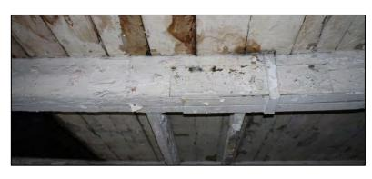
in the opposite face of the beam to the west (5/26), but not aligned, and also has a timber infill. A vertical compression scar in the face of the beam, immediately to the north may form part of the feature.
