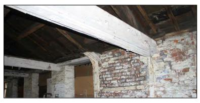
**Assessment of Significance:** These represent a repair to the decayed tie beam end, and are not thought to be early features, and are therefore considered to be of LOW significance.
