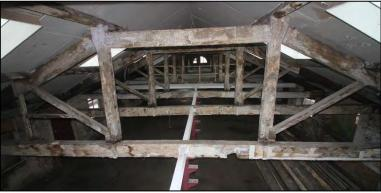
large scantling rectangular section, tenoned into the tie beam below floor level, with the joint apparently having been augmented subsequently with an iron stirrup. The jowled outer part of the foot of each queen post supports a slender straight brace to the principal rafter, itself tenoned into the jowled head of the queen post, that clasps the upper of three purlins to each pitch. Straining beams complete the truss, placed level with the head of each principal rafter.
