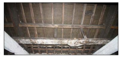
typical late 19<sup>th</sup> century or later style. A Baltic timber mark observed on the foot of one rafter (*5/71*) suggests that all are of imported European softwood. Similar-section timbers were also added as collars to most rafter pairs from Bay 3 eastwards, for the insertion of a suspended ceiling, almost certainly undertaken at the same time.
