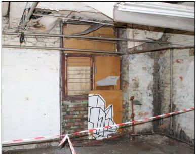
visual evidence for the installation of fire protection during the early 20th-century. Given that the original sprinkler system (5/07) has been removed, this feature will represent the only internal evidence for this important upgrade of fire protection, and is therefore considered to be of MEDIUM significance.
