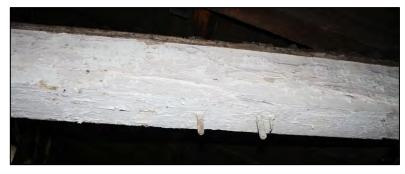
arrangement is typical of the attachment for J-shaped line shaft hangers, and the position relative to the long wall of the mill is also typical. However, little evidence for a shaft in this position was observed elsewhere on the 5<sup>th</sup> floor.
