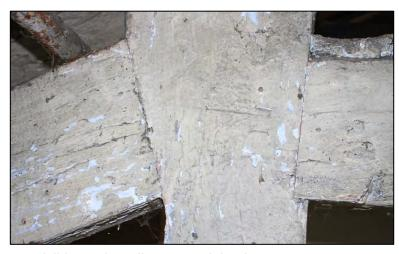
a corresponding assembly mark was visible on the adjacent straining beam.
