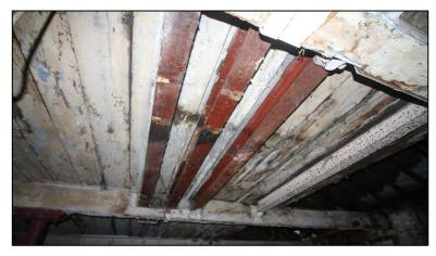
similarly carried on a cast-iron L-section bracket on the inner face of both tie beams. It is unclear whether the beams are associated with a bearing box above the window in the south wall (5/62) and with beam 5/60 to the south.
