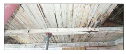
beams are jointed above the column head, comprising two members to each side of the beam. Several rolling stamps bearing the name of the Frodingham Iron and Steel Co were observed, demonstrating the beams to be of 20<sup>th</sup> century date, and almost certainly associated with strengthening works to the eastern end of the roof structure undertaken during the installation of a new stair tower (*5/70*).
