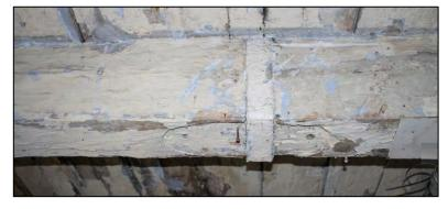
and is typical of a column headplate scar, possibly suggesting that there may have been an intention to replicate the two column rows seen on the floors below within the 5<sup>th</sup> floor. The scar is clearly covered by the stirrup between the tie beam and queen post of the truss above, demonstrating that the stirrups were not features of the original trusses, but were added subsequently.
