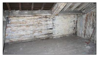
probably represents a later remodelling of the roof space either enclosing previously open eaves, or replacing damaged lath and plaster. However, it would appear to be a relatively early intervention given the similarity with the white and Dolly Blue paint layers also observed on the original roof trusses (6/01) and purlins (6/02). The eastern two bays of the northern eaves also retained planked rather than plaster eaves partitions.
