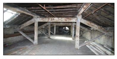
trenched into the principal rafters. All are butt jointed above each truss.
