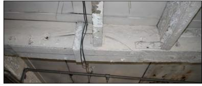
the beam and the stirrup to the queen post above, suggesting that there was significant damage to the beam to allow the plates to be manoeuvred into position.
