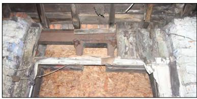
also been cut to accommodate the feature, which probably housed a rail for an external hoist
