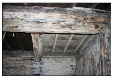
on an iron bar that lapped over the straining beam of the adjacent trusses, and has a Baltic timber mark (6/24) on its northern face, demonstrating it to be of relatively early date.
