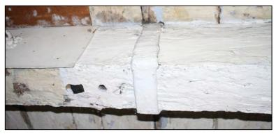
It has rounded ends, and is typical of a column headplate scar, possibly suggesting that there may have been an intention to replicate the two column rows seen on the floors below within the 5<sup>th</sup> floor. The scar is shallower than that to the south (*5/46*) but also covered by the stirrup between the tie beam and queen post of the truss above, demonstrating that the stirrups were not features of the original trusses, but were added subsequently.
