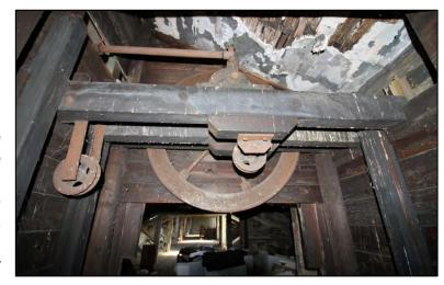
and affords access into the hoist tower, which retains timber framing carrying a large pulley wheel, and two smaller pulley wheels for a rope on the western side. The aperture between floors (*5/14*) also has an *in-situ* cover.
