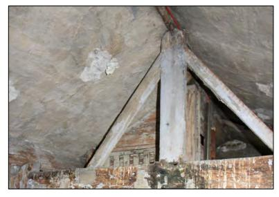
eastern side by additional support for the ridge board (6/13), possibly suggesting that the roof below the plaster retains its original layout.
