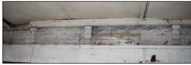
end of the ceiling planks of Bay 12. The northern end of the beam is chamfered to the wall face, providing slight architectural detailing, but the members are joined with a simple scarf joint, and a butt joint, the latter possibly representing the attachment of a replaced member.
