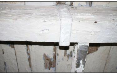
part of the bay. This does not have rounded ends, like others seen at this end of the mill, and has a square socket cut into the east face of the beam above.
