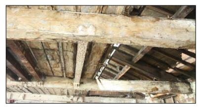
probably replaced an earlier timber example. Appears to be associated with a bearing box above the window in the south wall (5/62) and with three similar beams to the north (5/61).
