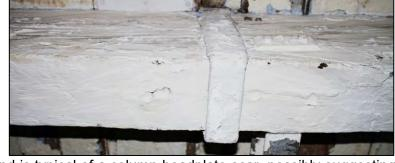
the bay. It has rounded ends, and is typical of a column headplate scar, possibly suggesting that there may have been an intention to replicate the two column rows seen on the floors below within the 5<sup>th</sup> floor. The scar is covered by the stirrup between the tie beam and gueen post of the truss above, demonstrating that the stirrups were not features of the original trusses, but were added subsequently.
